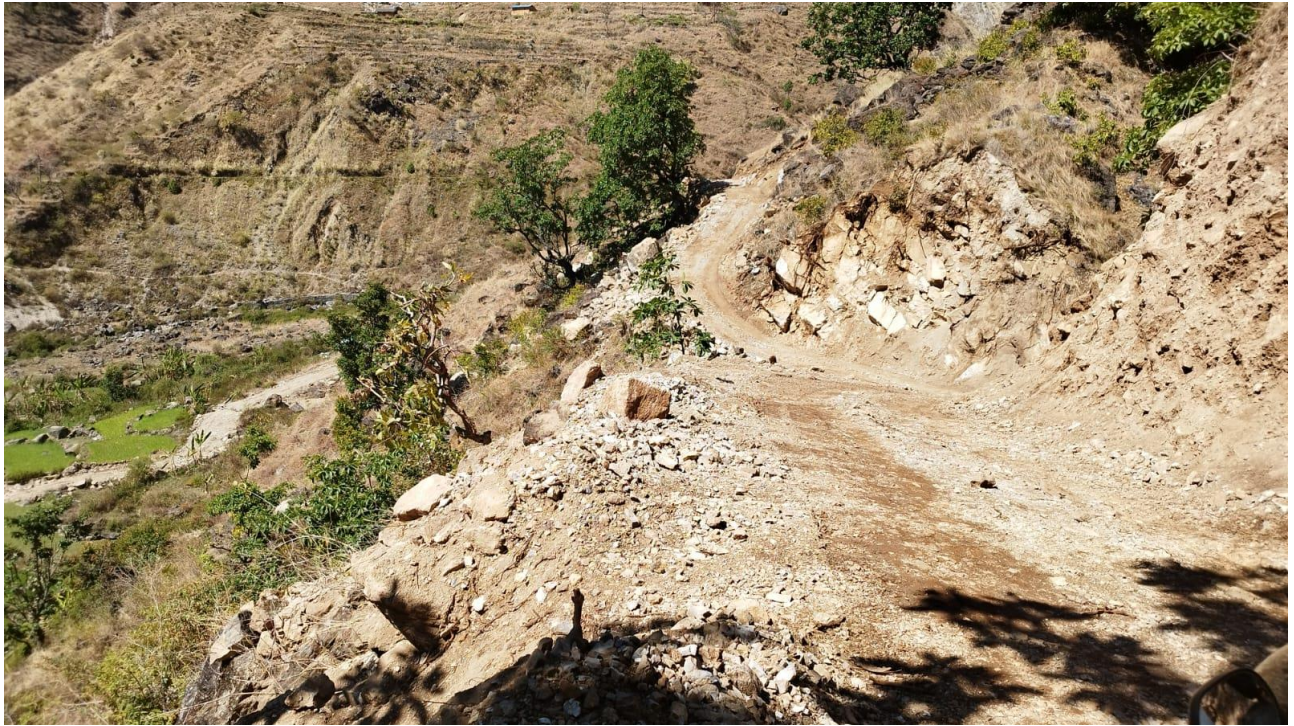
Excavation works for track opening at AB8.
