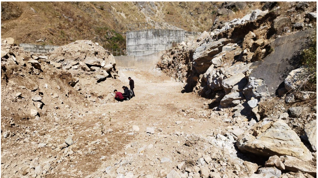
Excavation work of Settling basin, Intake.
