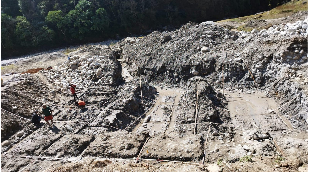
During laying of Earth Mat in powerhouse.
