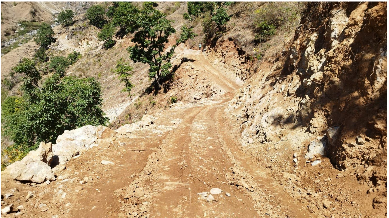
Excavation works for track opening at AB9.
