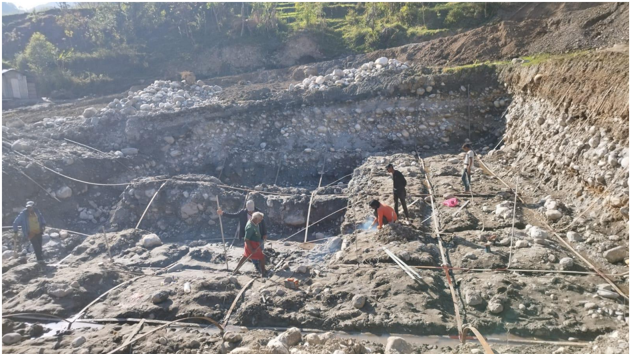
During laying of Earth Mat in powerhouse.
