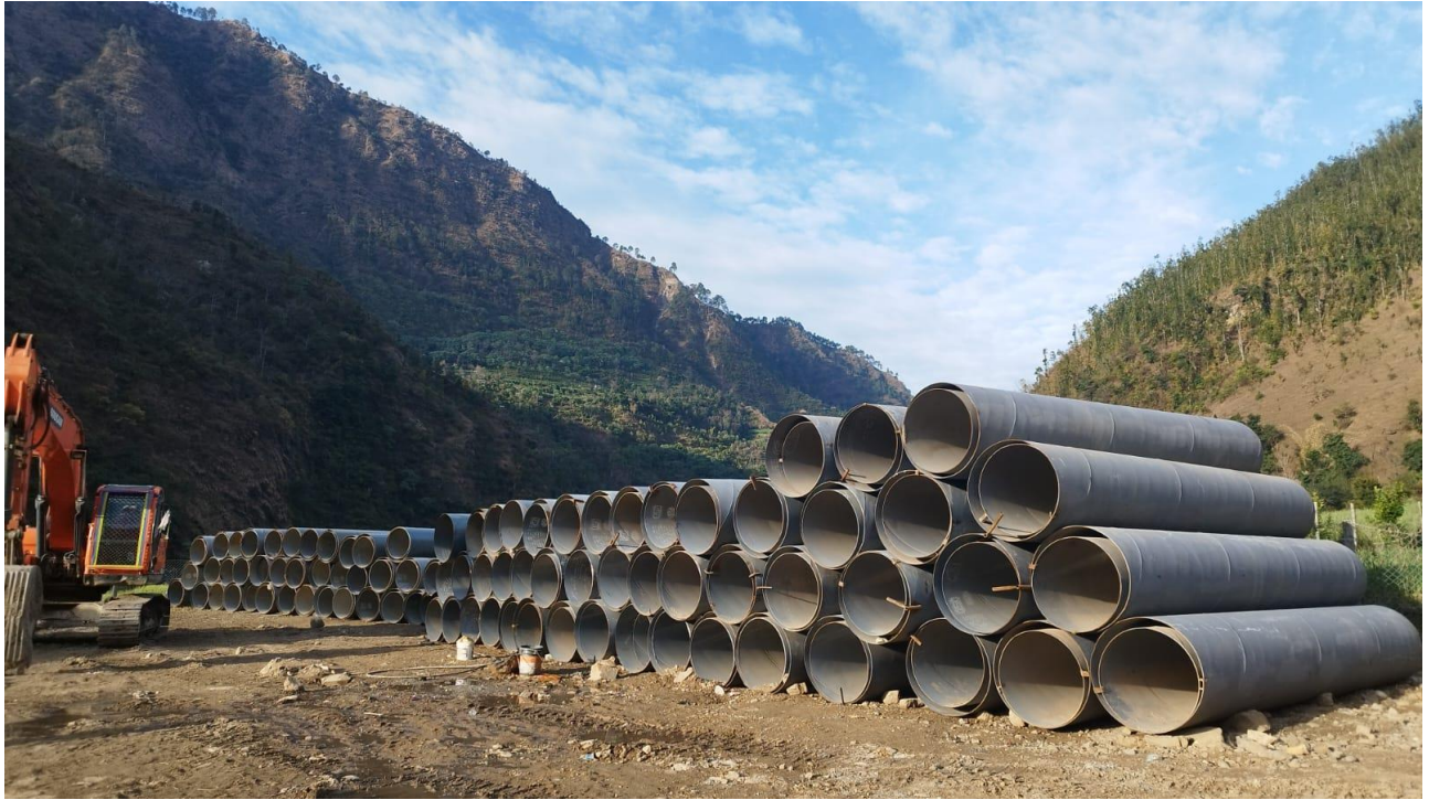
Pictures of pipes received at site in the yard
