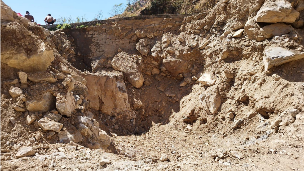
Excavation work of Spillway.
