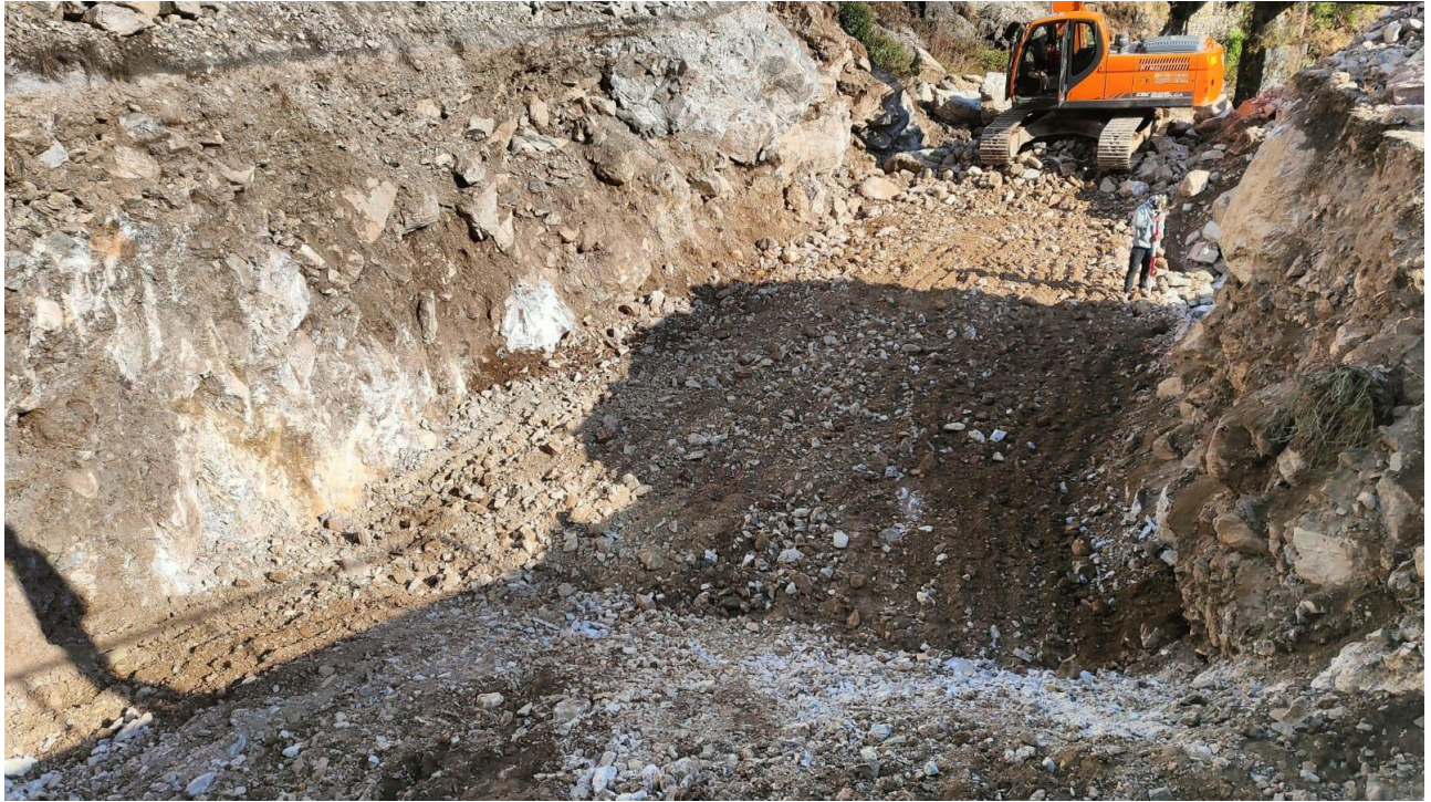
During excavation work of settling basin.
