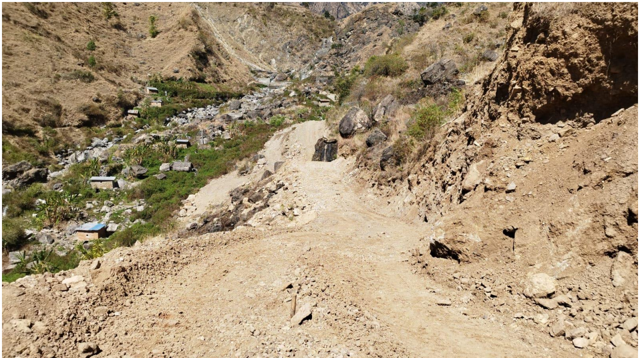
Excavation works for track opening at AB5.
