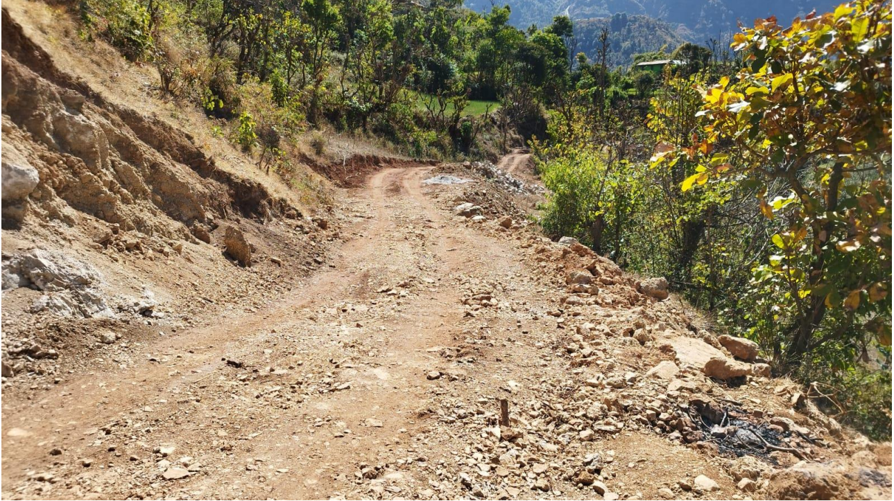
Excavation works for track opening at AB15.
