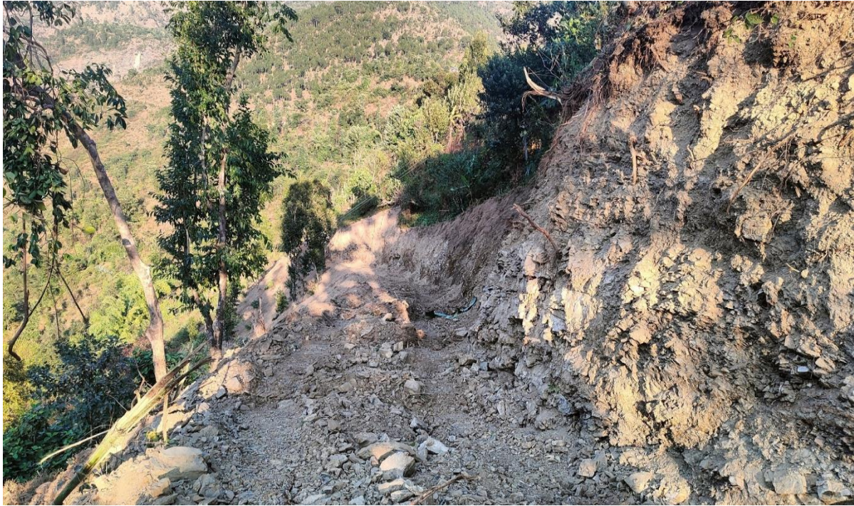
During excavation works for track opening.
