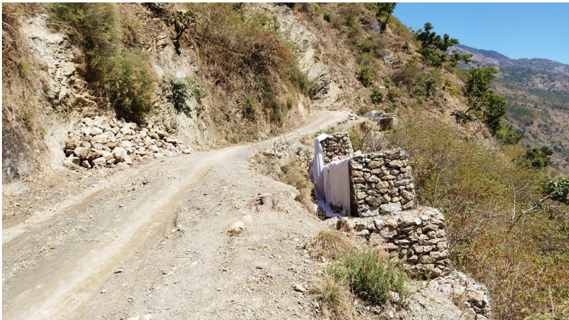
Protection works of access road for extra widening.
