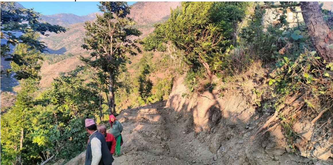
During excavation works for track opening.
