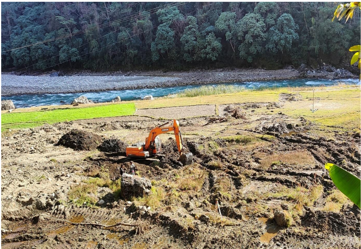
During excavation of machine foundation at level 929.295.
